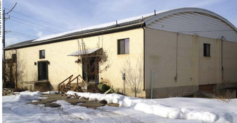
The new Logan church will require major renovations.
