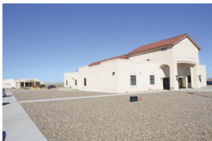
The new Gila Mountain church is situated in the foothills of Yuma, Ariz. The former church, in the rear, will be used as a fellowship center.
