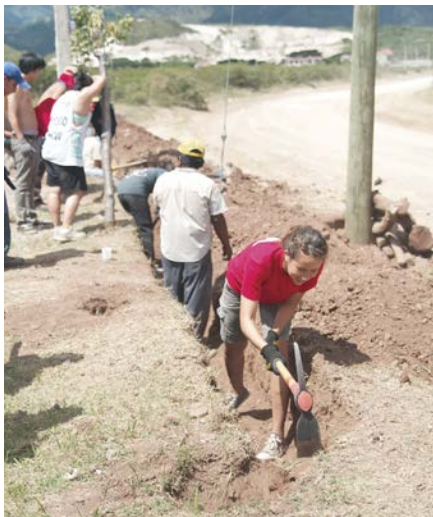
The construction team worked long hours in the hot Honduran sun.
