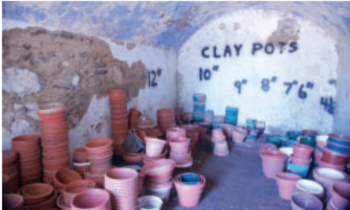
Today the vault at Battle Creek's Oak Hill Cemetery is used to store pots.
