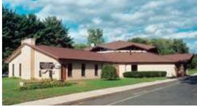
The construction of Hope church took place during the winter and spring of 1993. The octagonal sanctuary is flanked by a fellowship hall on one side and classrooms on the other.
