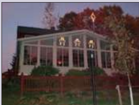
Construction on a sun/worship room for the members of the South Berwick Fellowship group was recently completed.
