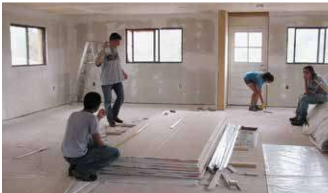
Students learn to measure and cut wallboard for both walls and ceilings.
