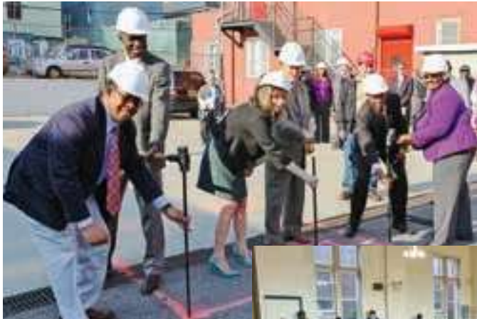
School and conference administrators participate in a groundbreaking ceremony for renovations at the Greater New York Academy.
