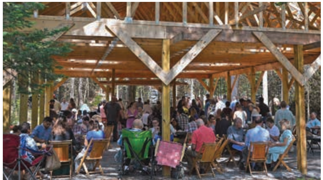
After the church service, annual meeting attendees gathered for lunch under the newly-constructed pavilion, built to serve as a picnic area for tourists drawn to the Sabbath Trail and church.
