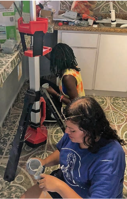
Volunteers help to repair a home damaged by Hurricane Maria.
