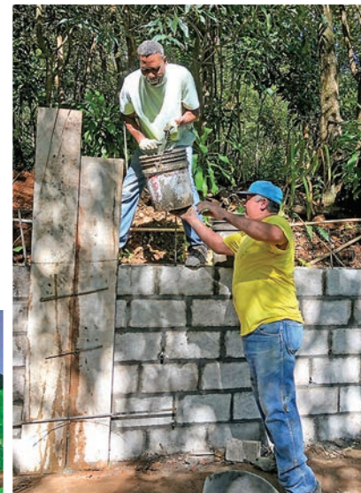
Workers help to build a retaining wall.
