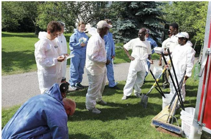
Volunteers gear up beside the ADRA Response trailer to tackle flash flood damage in Chestermere, Alberta.
