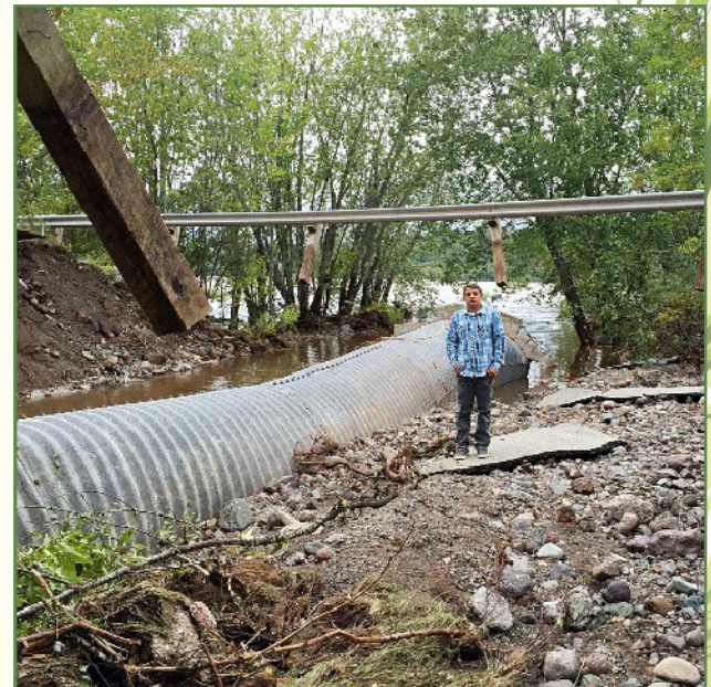
In the light of day, Ricky poses where an entire section of highway was swept away along with their car. Note the guard rail and posts dangling in mid-air!
