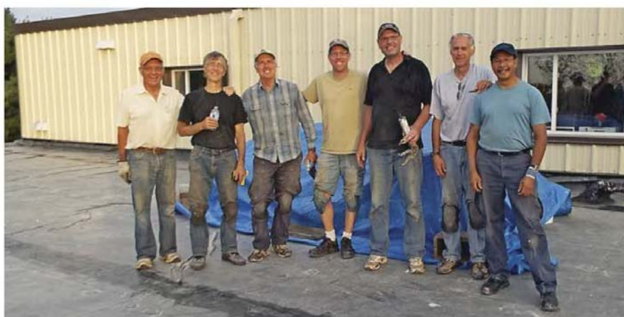
Kevin Scott (3rd from right) heads up the team of volunteers that replaced the roof at Sandy Lake Academy.
