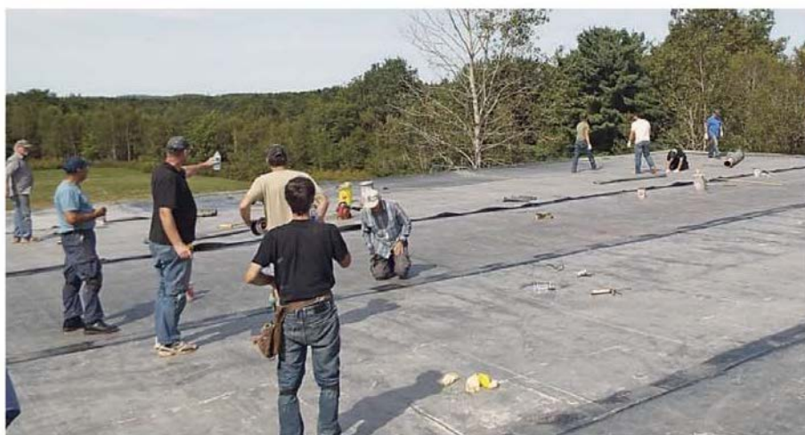
Volunteers installing the new EPDM rubber roof at Sandy Lake Academy.
