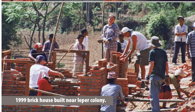
1999 student Shad Lehmann building at the house.
