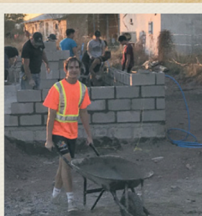
Kingsway students begin construction of a church building in Tesopaco, Mexico.
