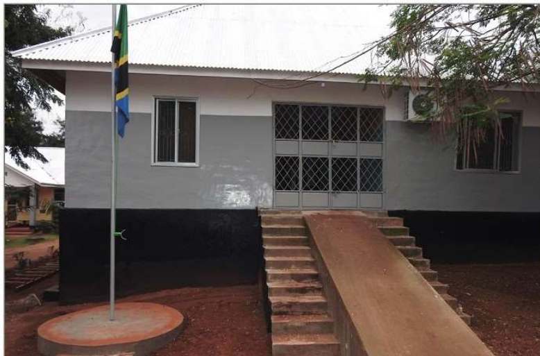
Mombo Health Centre's newly renovated exterior and interior.
