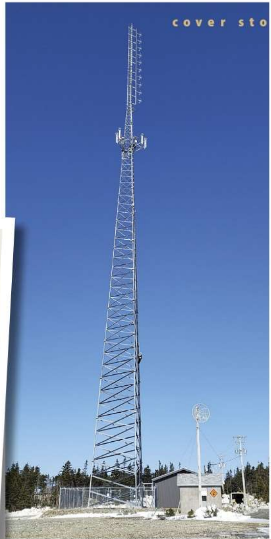
The tallest free-standing structure on the island of Newfoundland, is the 350-foot, 100,000-watt Lighthouse FM tower.
