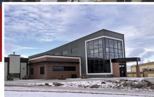
New library nearing completion
