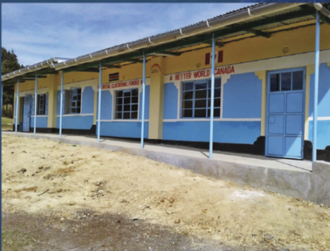
Recently completed special needs classrooms at Huhoini Primary School, Kenya
