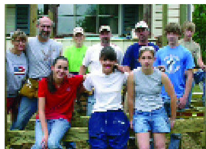
These Hanover church members and youth pause from building a wheelchair ramp and doing other jobs for a local senior citizen.
