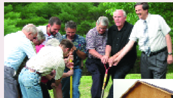
Conference officers help break ground for the new youth chapel being built at the Valley Vista Adventist Center in Huttonsville, W.Va.
