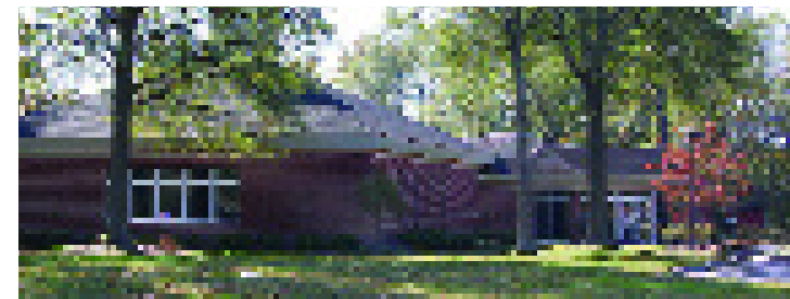
Redeeming Grace Fellowship now miraculously worships rent-free at this new location, a gift from the owning congregation.
