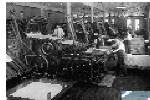
Above: In 1921 the Review & Herald Publishing Association presses could produce between 1,500 and 1,800 impressions per hour (IPH). Right: Today the Harris M-300M 6 unit web press can run the Visitor at an average 36,000 IPH and uses approximately 1,140 feet of paper per minute.
