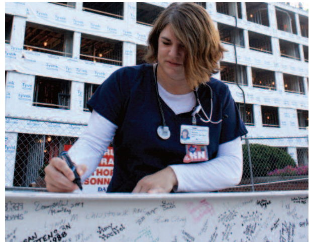
Michelle Romano, RN, from Kettering Medical Center’s Emergency Department, signs the last steel beam for the new Ben and Marian Schuster Heart Hospital.
