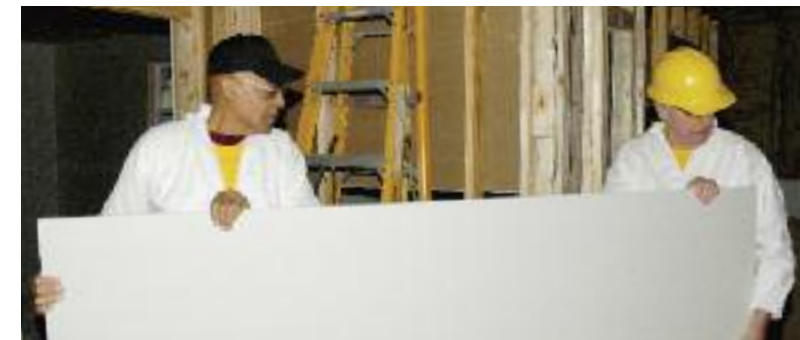
Eldred Pritchett and Mason Craig move drywall.
