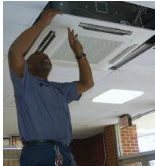
A workman installs the school's new $800,000 heating, ventilation and air-conditioning unit.
