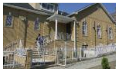
The remodeled front entrance to the Newark Spanish church.
