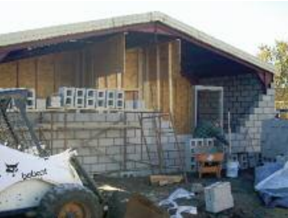
Walls go up in the New Horizons Community Learning Center.
