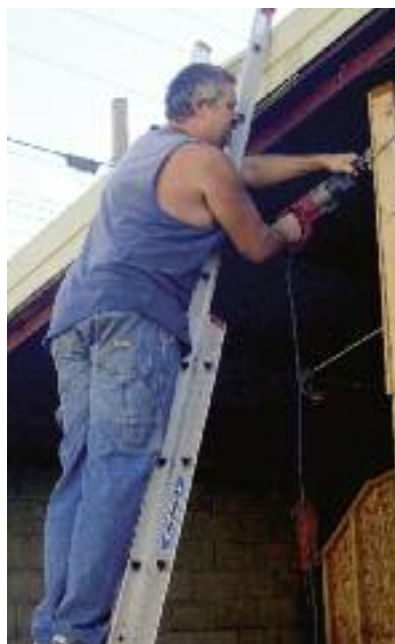
Volunteer Joe Kriner is hard at work on the renovation.
