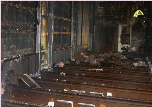
Fire investigators believe the fire that destroyed the sanctuary on February 21, 2012, originated in the electric organ.
