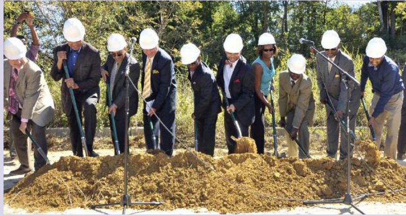
Leaders from the conference and Restoration Praise Center ceremoniously break ground on their new church building.
