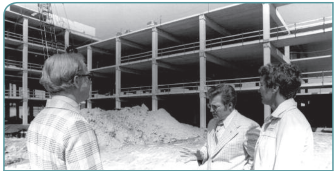
Elliott Fortner on the construction site of Sycamore Hospital
