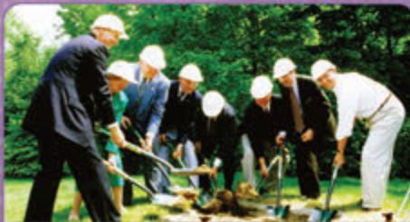
Construction begins on 100-bed Sycamore Glen Nursing and Rehabilitation Center on the Sycamore Medical Center campus
