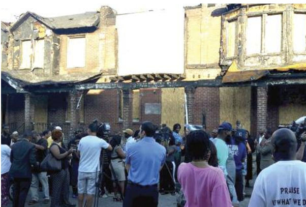
Community members survey the damage after the fire.
