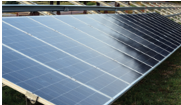
Highland View Academy's solar panels will supply electricity to the school.
