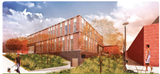
Architectural rendering of the new Gail S. and Bruce E. Boyer Health Professions and Wellness Center.
