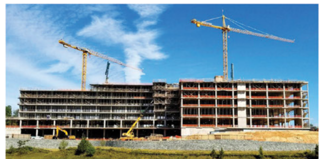
Construction in November 2017
