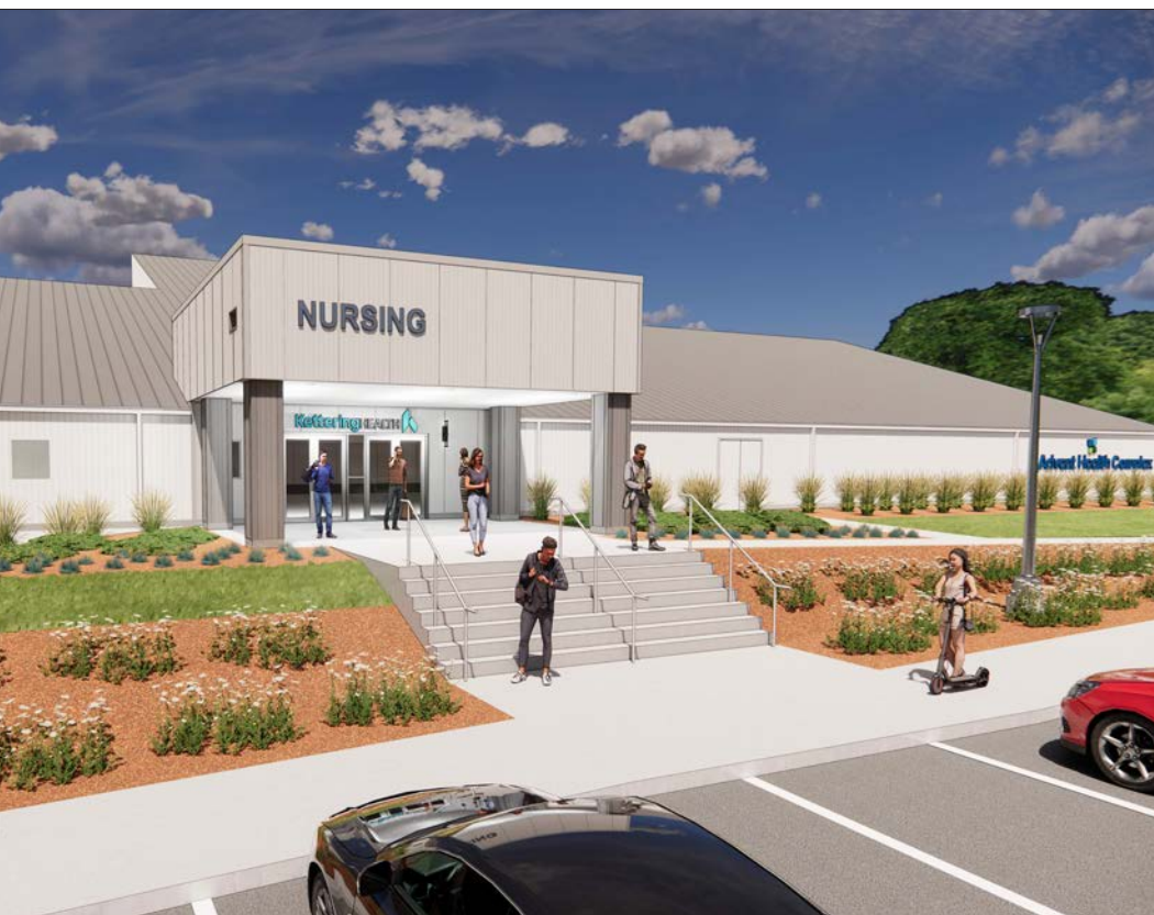
The Nursing Program will receive mobility-accessible entrance facing the south parking lot.
