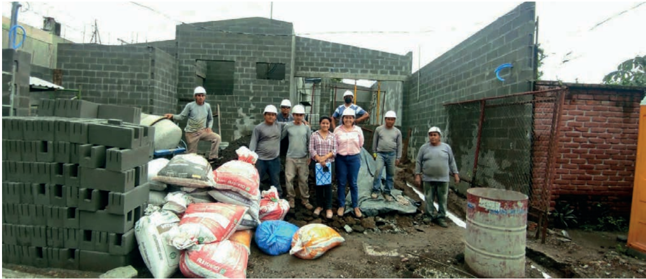
Architect Benavides and her daughter overseeing construction.
