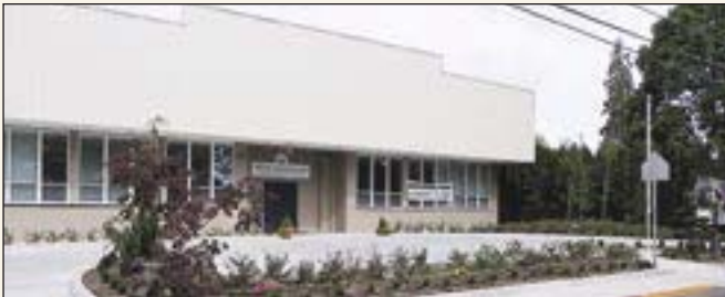
The McMinnville Adventist Christian School building, before and after its roofing and remodeling
