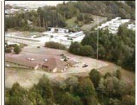
This aerial view shows the location of the radio tower near the Coquille Church.
