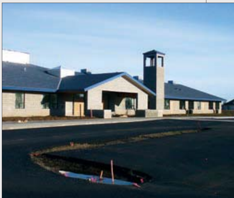
The almost-completed Rogers Adventist School in College Place, Wash.
