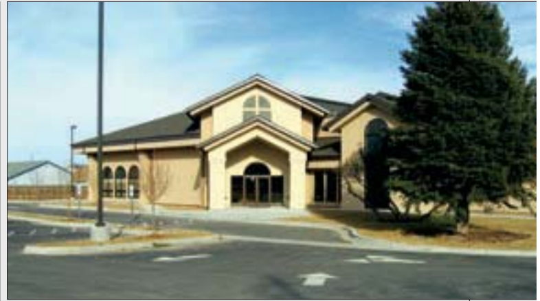
The 25-year-old Kuna congregation has just completed a sanctuary construction and facility remodel.
