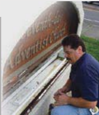
Brad Carpenter contemplates lighting issues during the church signage repair.
