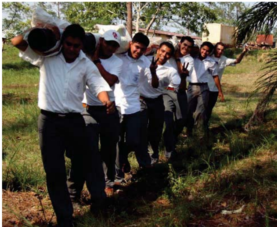
Happy to help, students from ICAP haul the 20-foot, 460-pound well casings to the well-drilling site.
