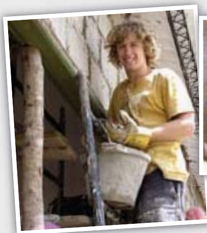
Paul Curtis works hard to patch up the spaces between the bricks and the roof.
