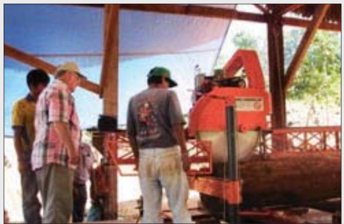
Cedar Creek/Woodland Church members purchased, shipped and set up a saw mill in Peru to aid in the construction of churches and schools.
