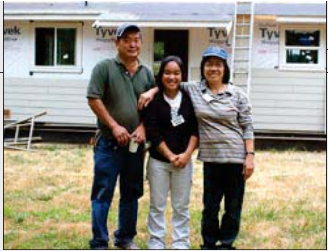
Pablito, Belma and Michelle Reyes praise God for their new Habitat for Humanity home in Poulsbo. SAGE volunteers helped to frame the house.
