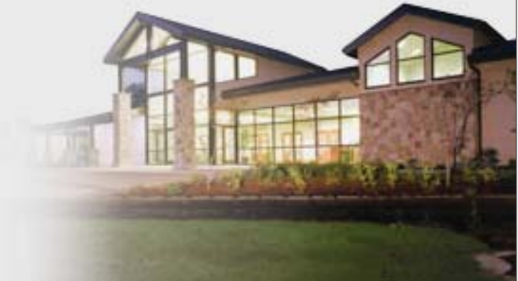
The Holden Convention Center, on the campus of Gladstone Park Conference Center, is serving as the temporary administrative headquarters for the Oregon Conference.
