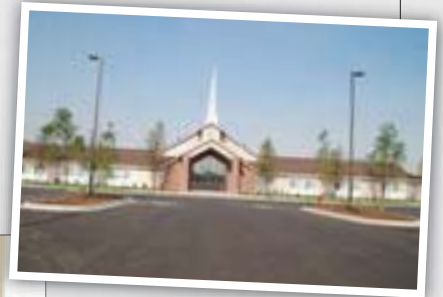
The new Meridian Church is complete with landscaping, parking lot and sanctuary.
