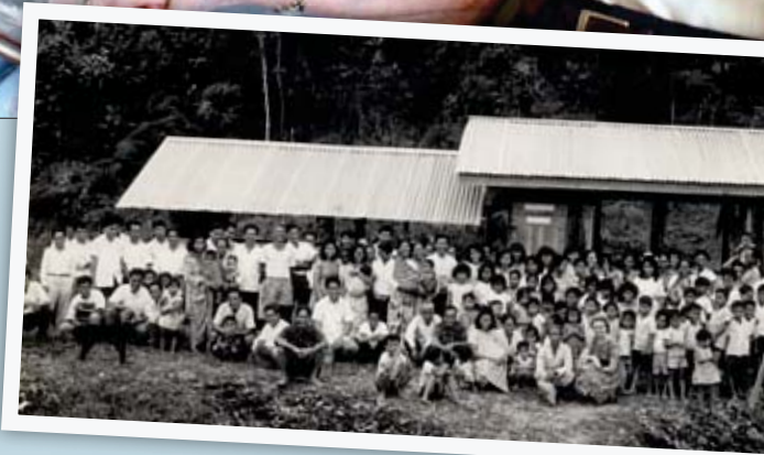
Located in the Sabah area of Borneo, these church members built the very first Lamb Shelter.
