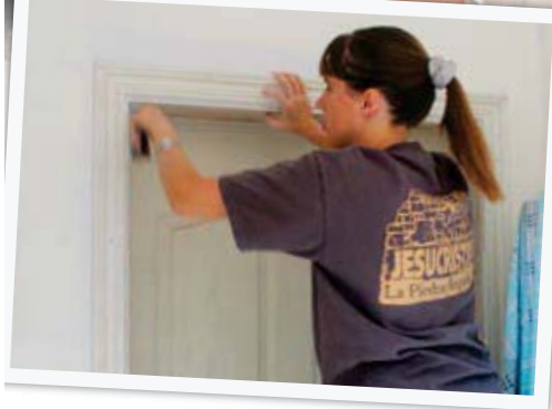
Sanding the door trim is boring work but was a necessary step before painting.
