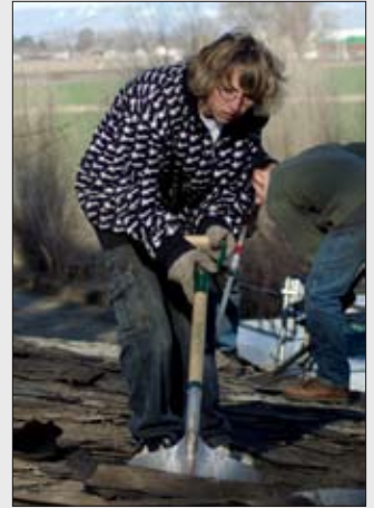
Jacob Larson strips a roof during the All Nations project.
