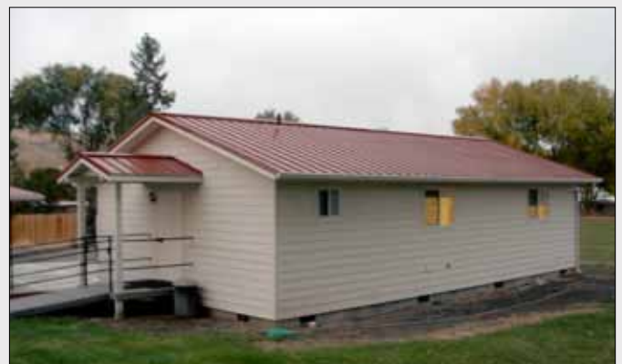
On the western edge of the Idaho Conference, the town of Dayville, Ore., enjoys a church plant valued at a replacement cost of more than $281,000.
